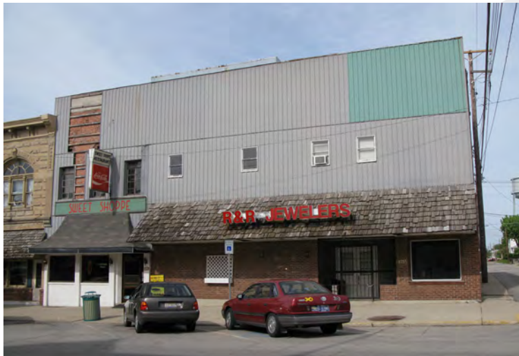
Unsympathetic alterations to this facade included metal siding that covered the original brick, an overbearing awning, and small windows that are unsuitable for the building size. (Not located in Remington)
